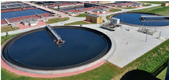
● Wastewater Treatment Plant in Wrocław
