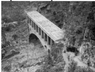
Fig.1 Conventional solution including a roof slab
