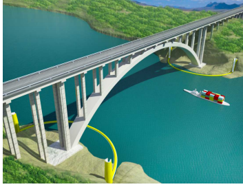
Fig.1 The effect drawing of anti-collision device
