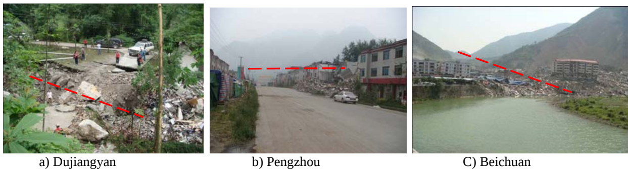
Fig.1 Buildings damaged due to fault propagate
